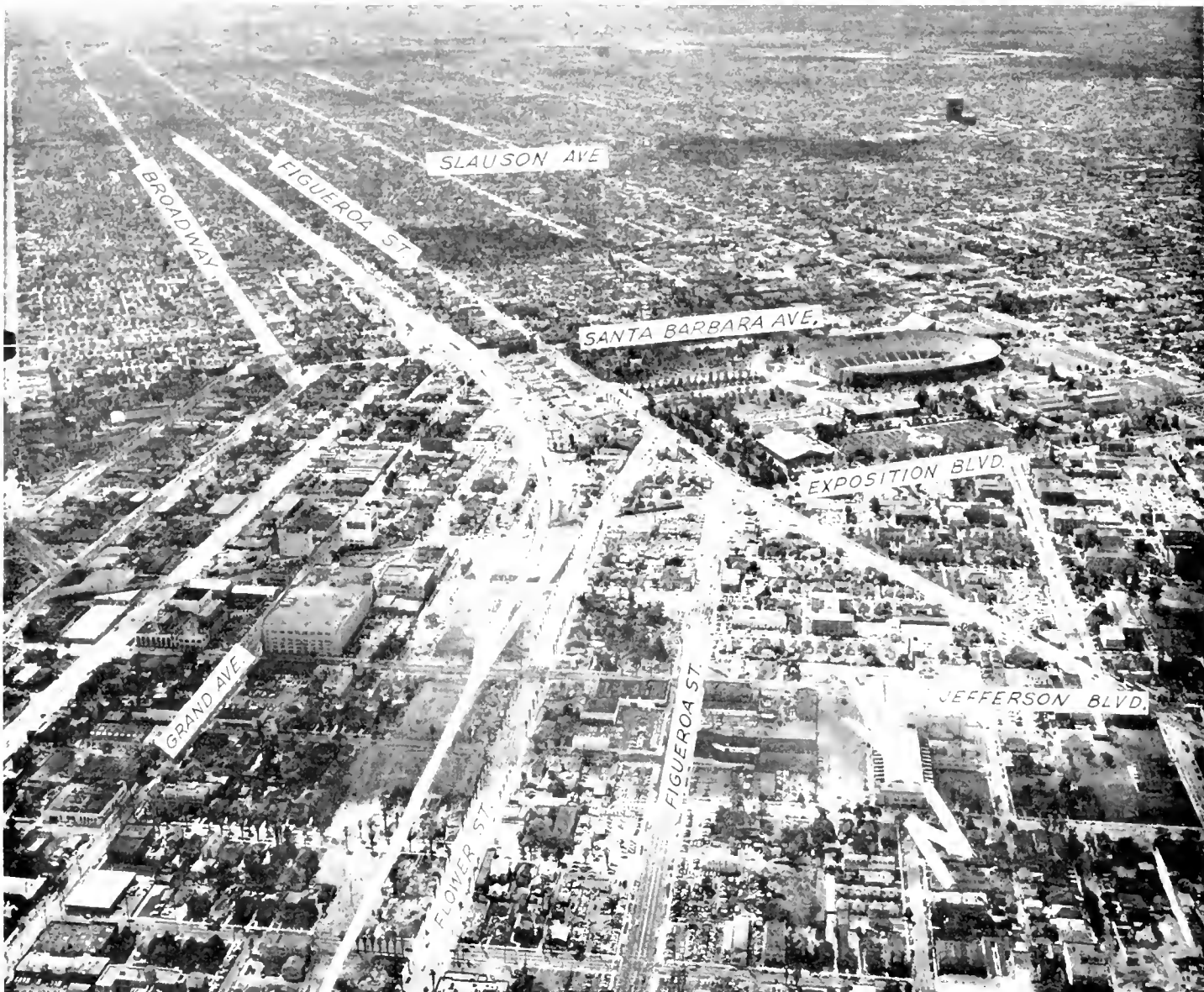
Looking southwesterly showing Harbor Freeway location close to Flower Street and Figueroa Street. Cleared right of way is in evidence foreground and center left. Los Angeles Memorial Coliseum in Exposition Park is shown center right.
